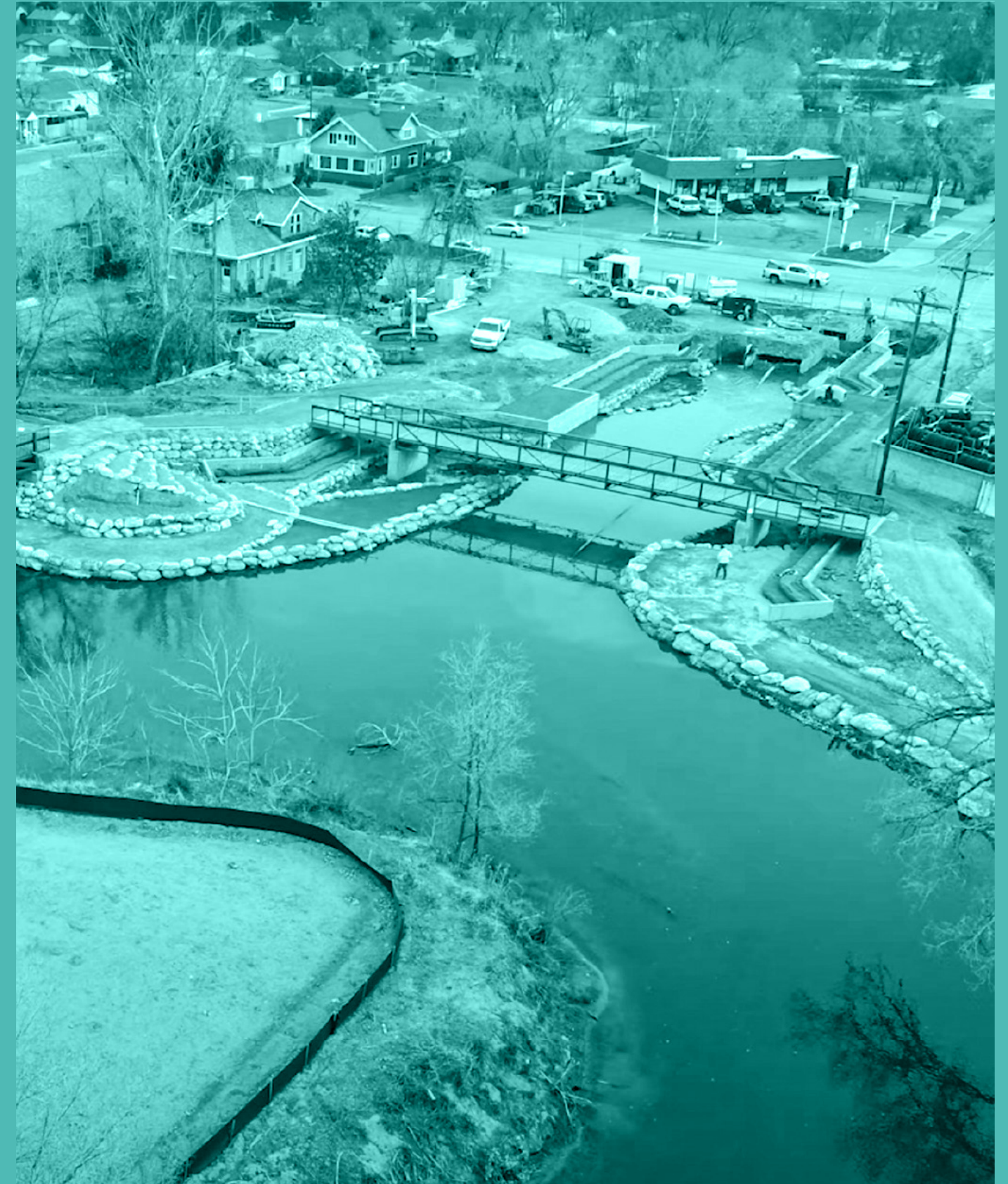
Figure 3: Daylighting of Red Butte, Emigration, and Parleys Creek at the Three Creeks Confluence in Salt Lake City.
