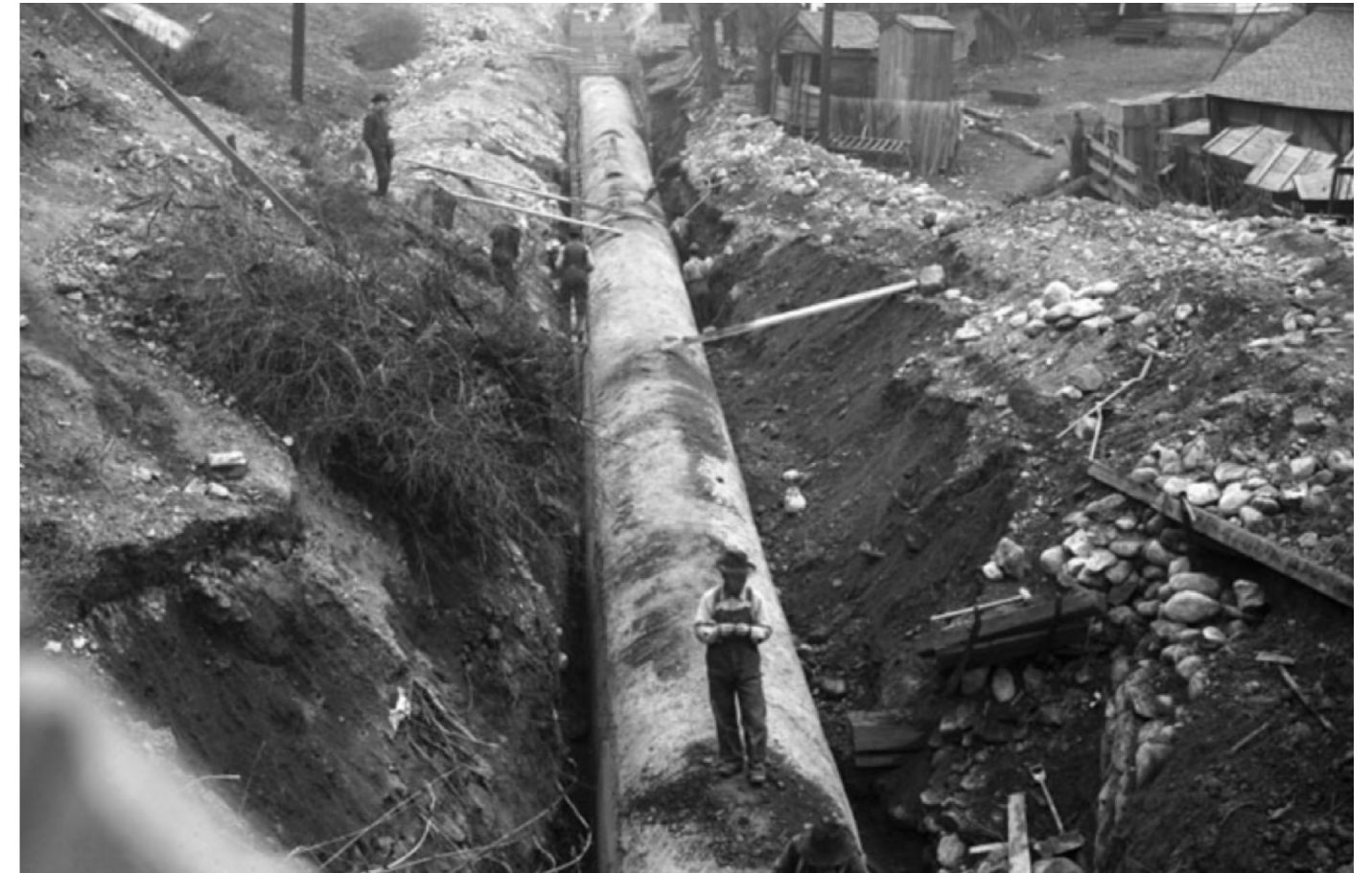
Figure 1: Burial of City Creek in culvert, circa 1910. Courtesy of Utah State Historical Society.
